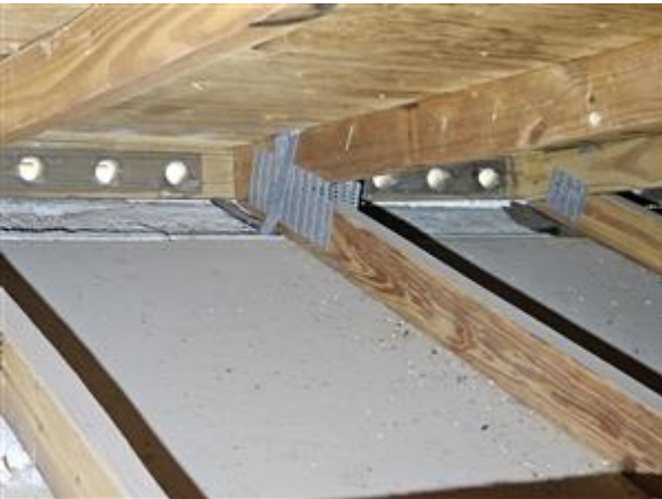
Roof to wall attachments(single straps)
